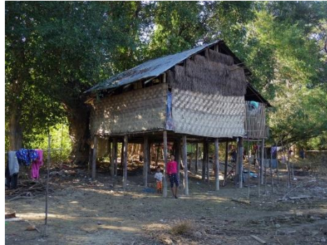
Rebuild bamboo house in Hinthada
