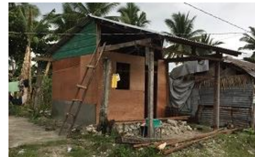
Rebuild bamboo house in Samar
